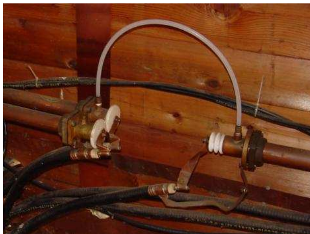
Figure 14.52: Flexible coaxial cables connected to rigid lines.
